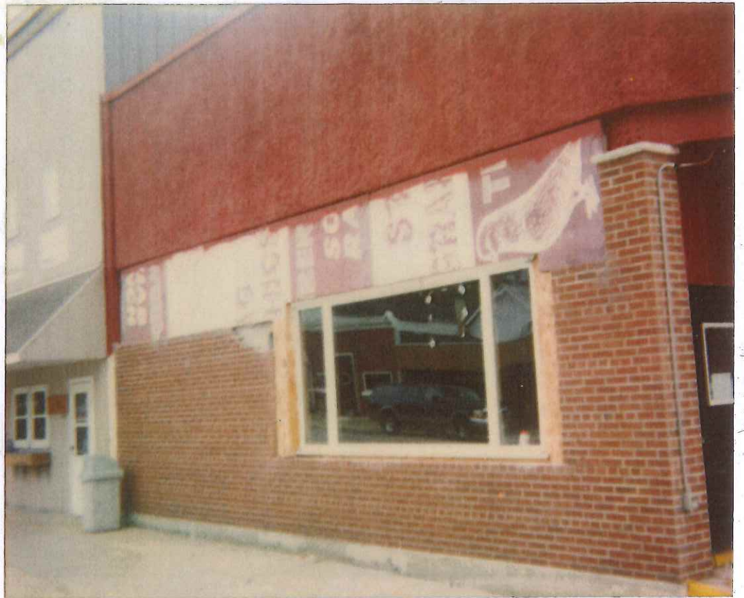
Yahr Building being painted Summer 2000
