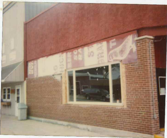
Yahr Building being painted Summer 2000
